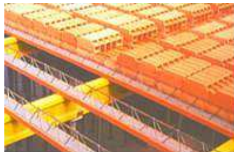
floor with precast beams
