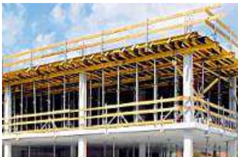
floor full concrete
